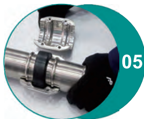
Position the clamshell over the sealing element, ensuring the lugs align with the grooves.
