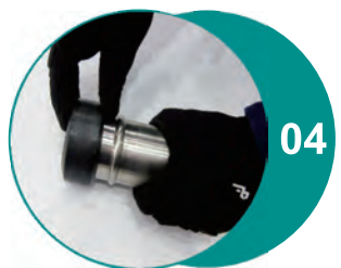
Insert the pipe ends into the seal to 2-3 cm on each side.
