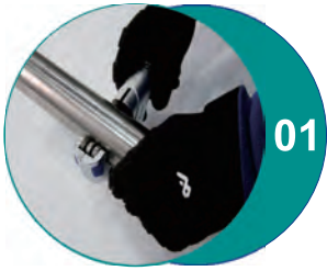
Use pipe cutter to cut the pipe.
