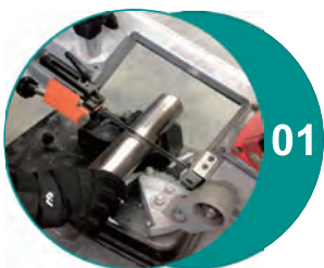
Use cutting machine to cut the pipe.
