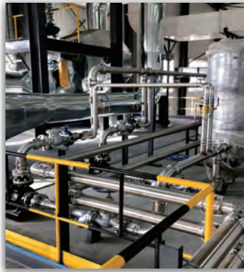
● Cooling water for new Material.
