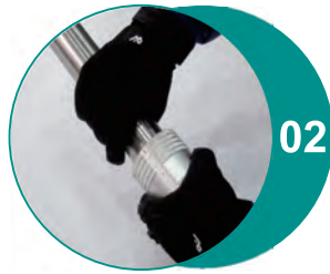
Deburr and chamfer the pipe end.
